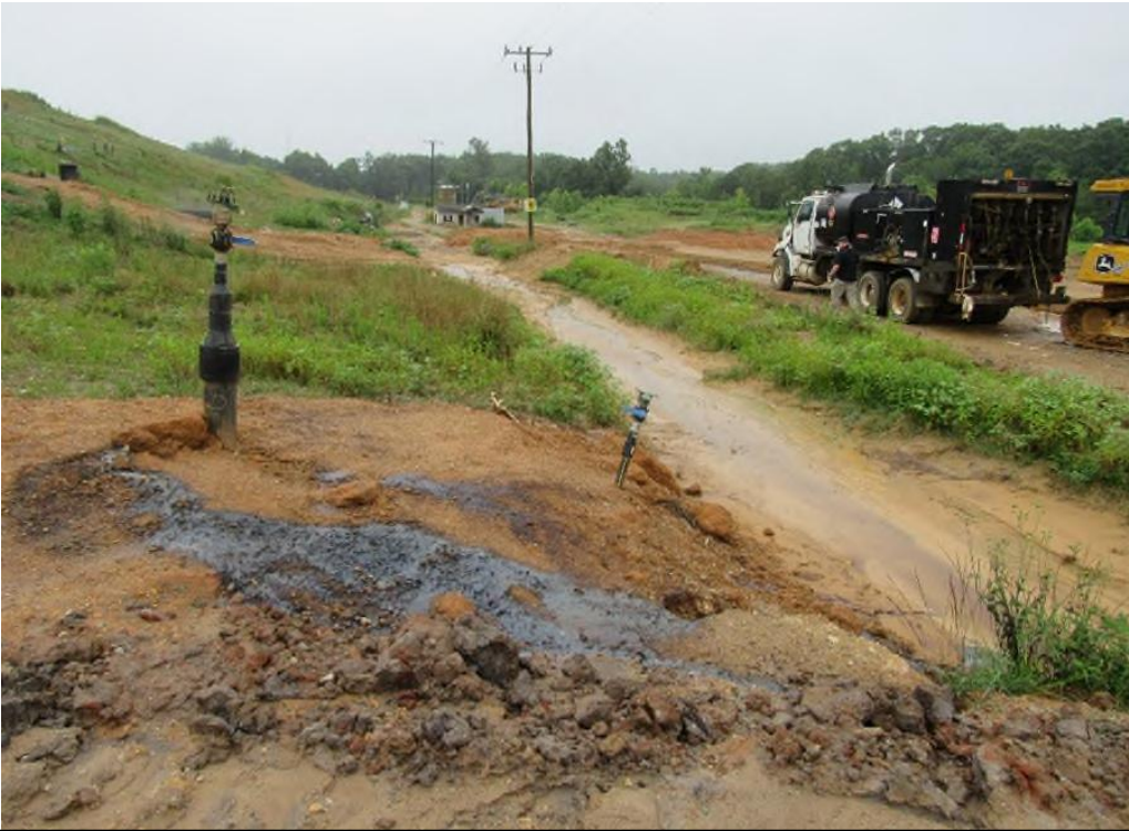
Site Name: Shoosmith SLF Permit# SWP587 Taken By: Jeremy Kazio and Andrew Peal Photo Number: 21 Date: 6/16/2025 Comments: Storm water ditch inundated with sediment
