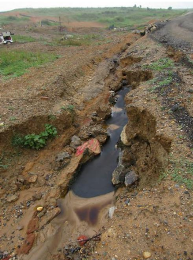
Site Name: Shoosmith SLF Permit# SWP587 Taken By: Jeremy Kazio and Andrew Peal Photo Number: 21 Date: 6/16/2025 Comments: Storm water ditch inundated with sediment
